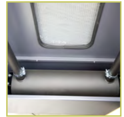
Residential muffler -35 dBA for enhance sound attenuation
