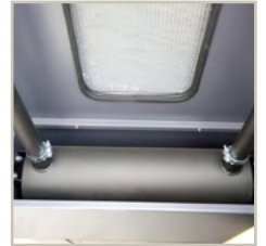
Residential muffler -35 dBA for enhance sound attenuation
